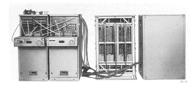
Telephone Central Office Set TC-2 is a complete, transportable, telephone exchange designed to handle local traffic, and originating and terminating trunk and tie-line calls in field wire systems serving corps and higher headquarters.
