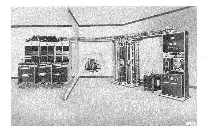
Telephone Central Office Set TC-10 is a complete, transportable, 270-line manual telephone exchange. It serves both local battery and common battery lines, and is arranged for handling, originating, and terminating trunk and tie line traffic.
