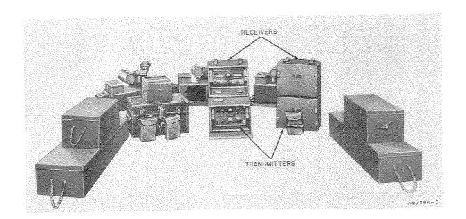
Radio Terminal Set AN/TRC-3 is a transportable, crystal-controlled, f-m, field, radio transmitting and receiving equipment which can be used in point-to-point, single or multichannel communication or as the terminal of a radio relay link in a system serving division and higher headquarters.
