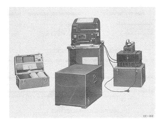
Teletypewriter Set EE-102 is a transportable field teletypewriter equipment used in weather reporting stations at division and higher headquarters, air fields, and stations of the Air Weather Command for communication of weather data.
