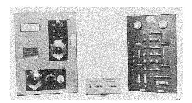
Emergency Radio Telegraph Transmitter TDK is a-m (mcw) equipment for emergency m-f transmission aboard ship. It provides a high degree of reliability, together with simplified operation and minimum drain from the power supply circuits.
