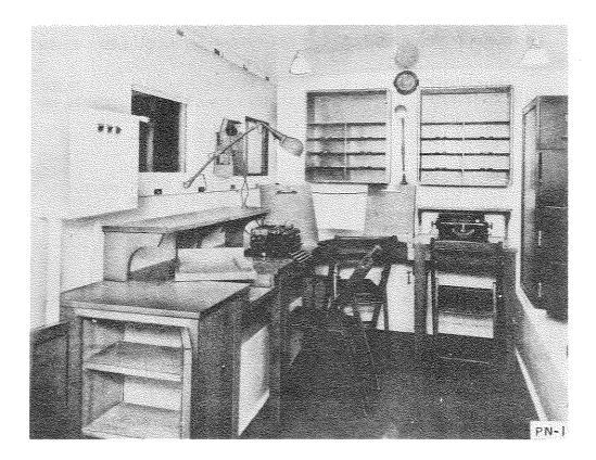
Mobile Coding Vans PN-1 and -2 are mobile operating shelters used at advanced-base cryptographic, radio receiving, or teletypewriter stations. These vans contain required office furniture, plus telewriter equipment. Provision is made for the installation of desired radio equipment.
