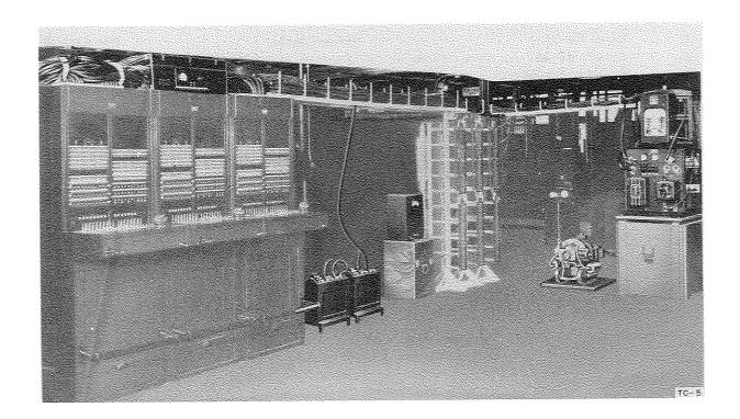
Auxiliary Telephone Central Equipment TC-5 is a group of installation components used to enable movement of Telephone Central Office Set TC-2 or TC-10 with a minimum of interruption of service at army or equivalent headquarters.
