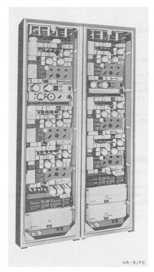
Carrier Terminal OA-5/FC is a six-channel carrier terminal equipment used to provide a maximum of 12 two-way, telegraph circuits on a four-wire basis, over type C or type H carrier facilities serving army and higher headquarters.
